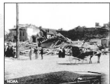
St. Louis tornado damage, May 27, 1896.
